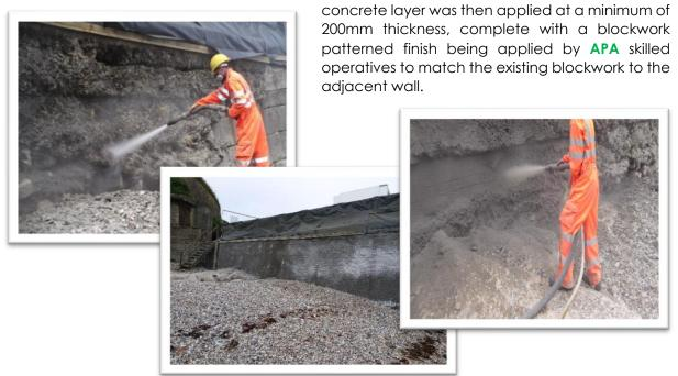
**The outcome:** Being the most efficient method of concrete application, the process of spray concreting the Southern face sea wall was completed in August 2016, ensuring this ever-popular destination could be promptly re opened to the public. The materials used for the
